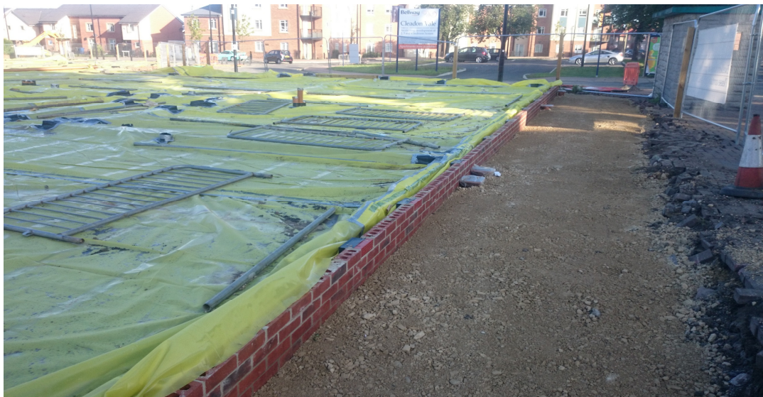
Photograph 3: Looking east at the eastern wing of the apartments.
